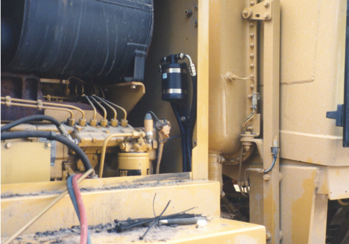
Receiver drier in place on forward engine wall.
